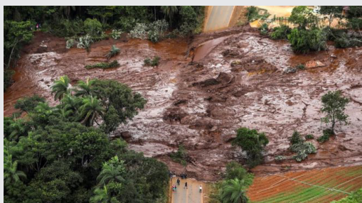
Figura 15 – The Vale dam disaster, 2019
